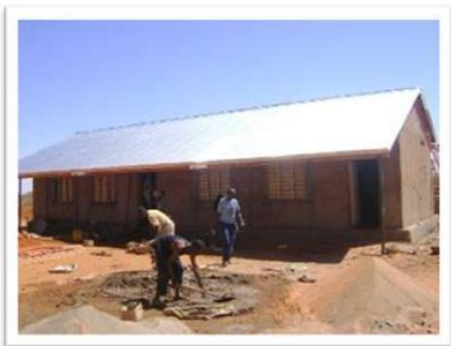
Primary School Extension under construction - Odweine
