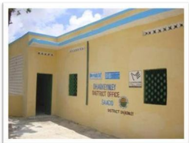
Dharkeynley District Office
