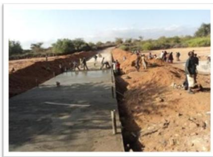
Construction of a drift in Hargeisa
