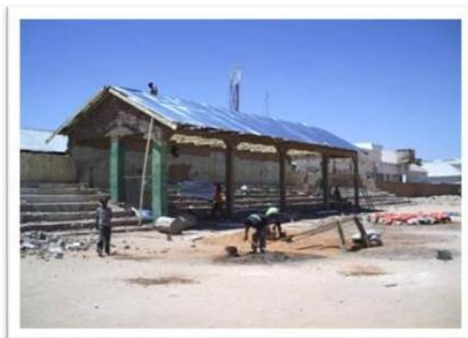
Galkayo Stadium Construction
