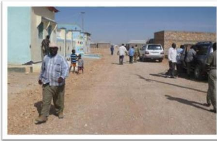
Bulsho Gravel Road after construction
