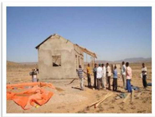
Health Post under construction Sheikh
