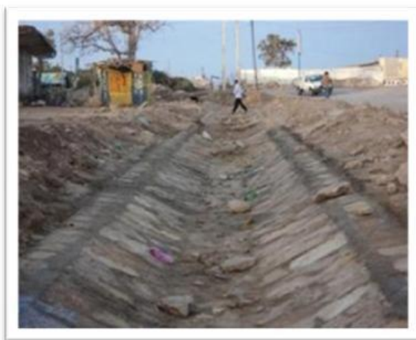
Construction of side drain in Berbera
