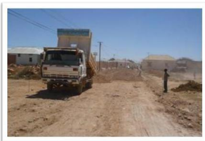
Hospital Road during construction
