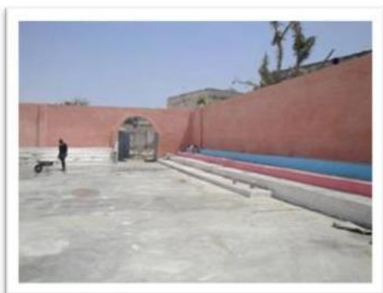
Hamarweyne Sporting Grounds construction
