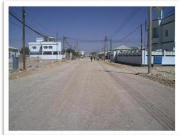
Gureye Gravel Road after construction
