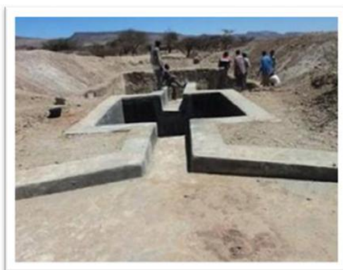
Construction of Berket in Borama
